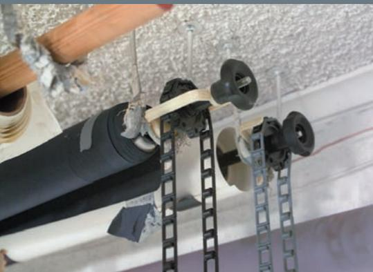
**Figure 2.** A Bogen, chain drive for raising and lowering seamless paper.
