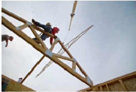
Installing a Truss © John H. Siskin All rights reserved
