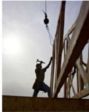
Hammering a Truss © John H. Siskin All rights reserved
