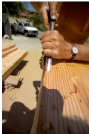
Gouging a Beam, original crop © John H. Siskin All rights reserved
